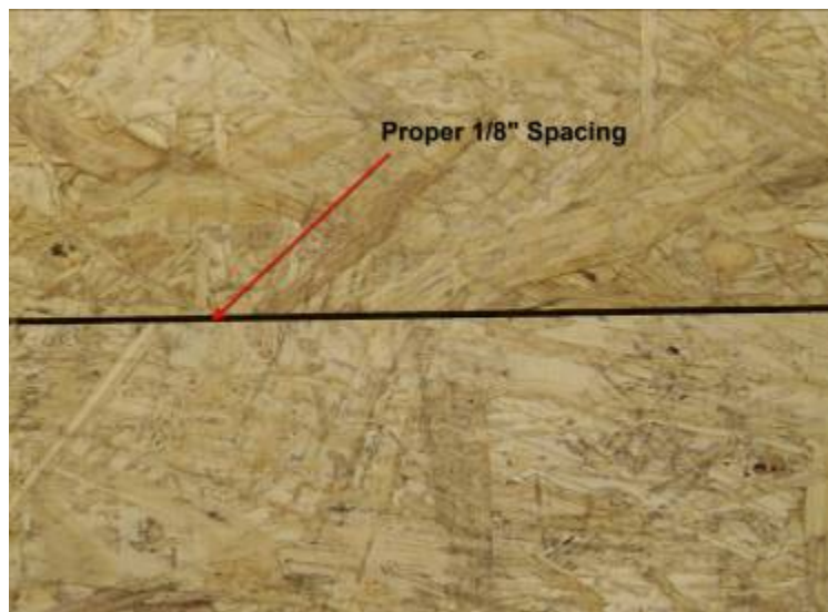
Correct installation of Advantech T&G Edge
